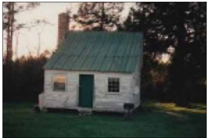
The original Coleman Homestead home before the addition and restoration.
