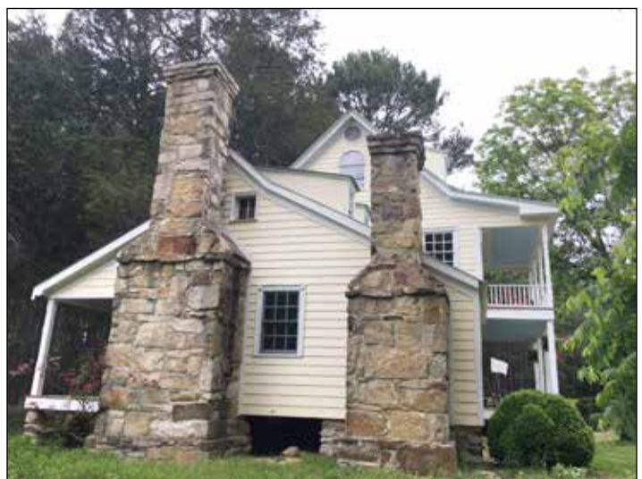
The restored house and original chimneys as seen today.
